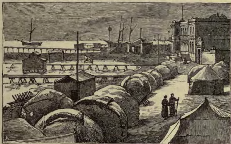
GOVERNOR'S HOUSE AND STORES AT KRASNOVODSK.
